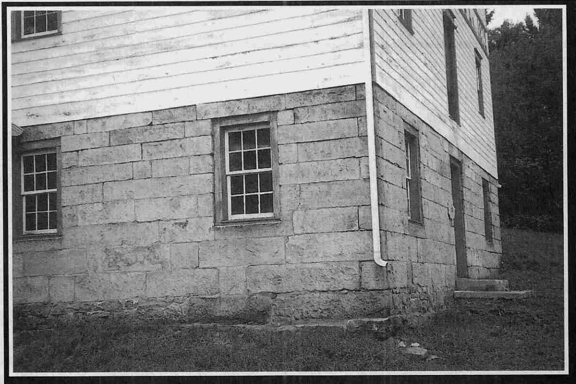
The Beachys were known for their stone cutting ability. They would drill holes in the rocks in the winter, put water in the holes, and expansion would break up the rocks. In the summer they used grain and water. These stones were cut, trimmed, and smoothed by Beachys.
