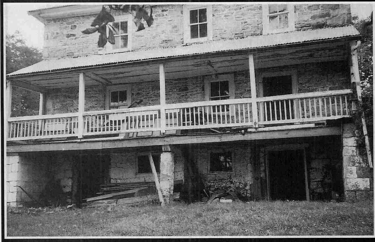
Notice short doorways into the basement.
