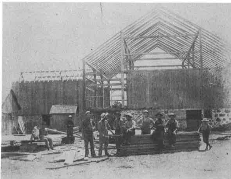
The barn being enlarged and rebuilt
